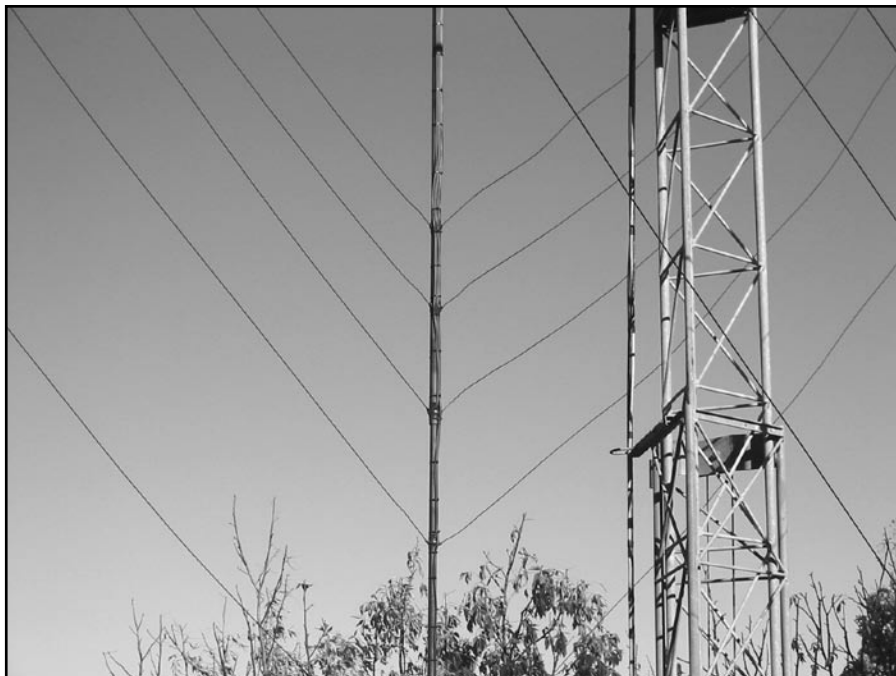
Figure 3 — Don't drill holes through your spreaders. Hold the wires in place on the spreaders and secure them with a piece of string. Then wrap the string with electrical tape and use a UV-resistant cable tie to keep everything in place.
