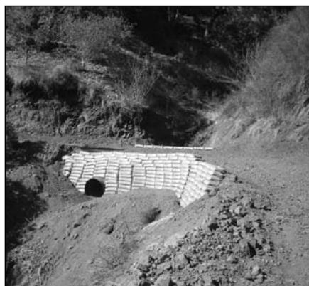
Figure 2 — A reminder of why one must consider ingress/egress problems
