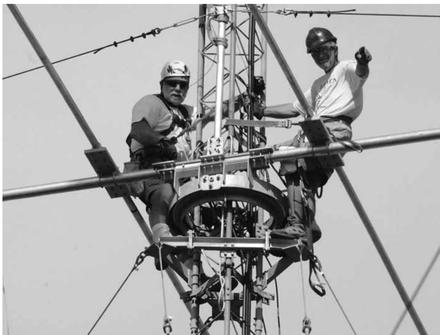
Figure 1 — W2GD and K4ZA install a 40 meter OWA at 185 feet at the NR5M super station.
