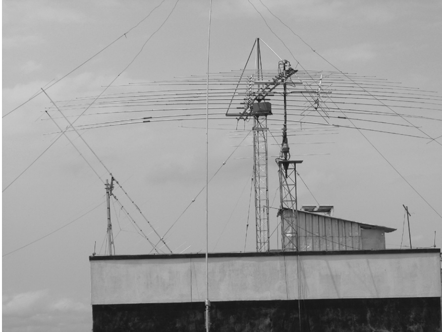
Antennas at ET3AA, featuring the large log periodic beam [K4ZW photo]
