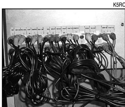
Figure 2 — The patch panel for the amplifier inputs
