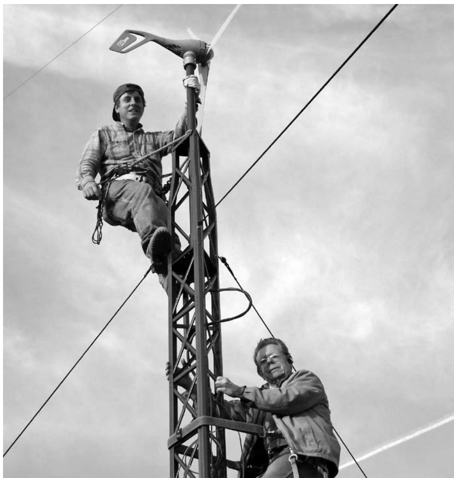
Figure 2 — K6XX (top) and K6HJU complete the Air Breeze installation.
