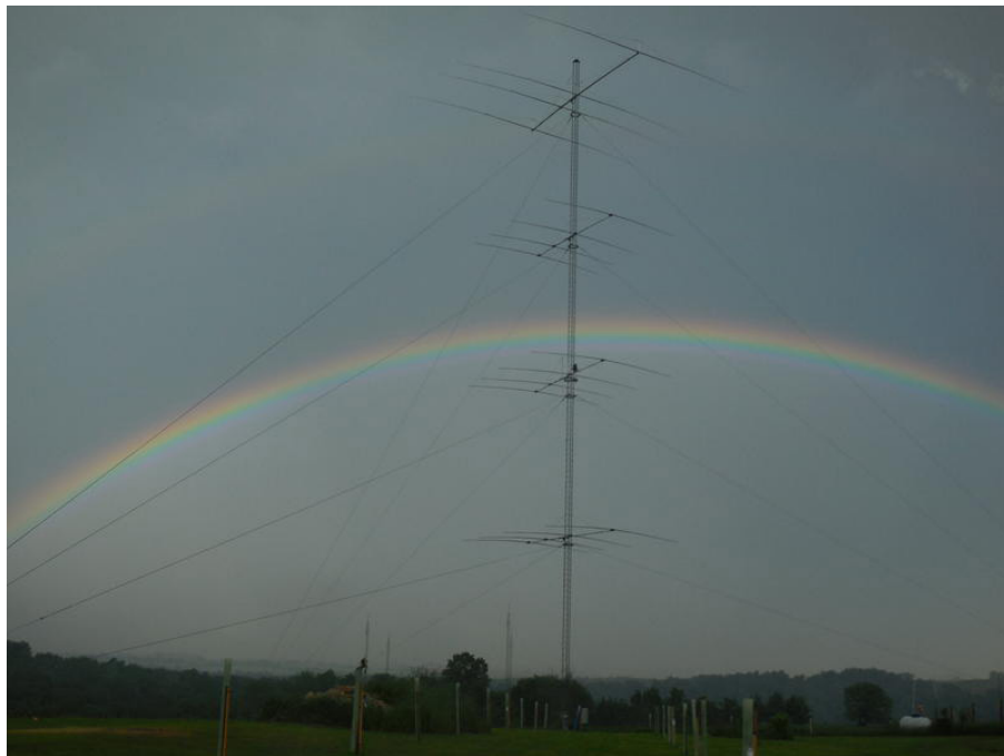
Figure 1 — The main tower — a 165 foot rotating Rohn 55G with full-size M 2 40 meter 40M4FS-125 at 156 feet with three 4 element SteppIRs at 112 feet, 76 feet (on TIC ring) and 40 feet. All guys are Phillystran. [Glenn Johnson, WØGJ, photo]
