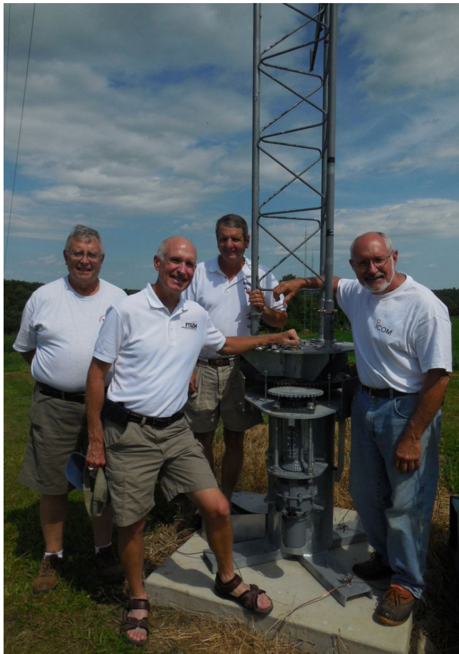
Figure 2 — The big tower has the KØXG rotating base and guy rings. The KØXG boom brackets are used for easy mounting of antennas. The prop pitch rotor is from Curt, K7NV. (LR) Richard, KØXG; Craig, K9CT; Roger, N4RR, and Glenn, WØGJ. [Glenn Johnson, WØGJ, photo]
