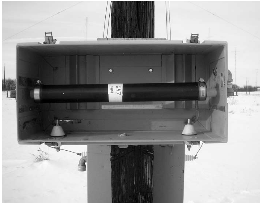
Figure 3 — 600 Ω noninductive terminator used at the far end of each rhombic
