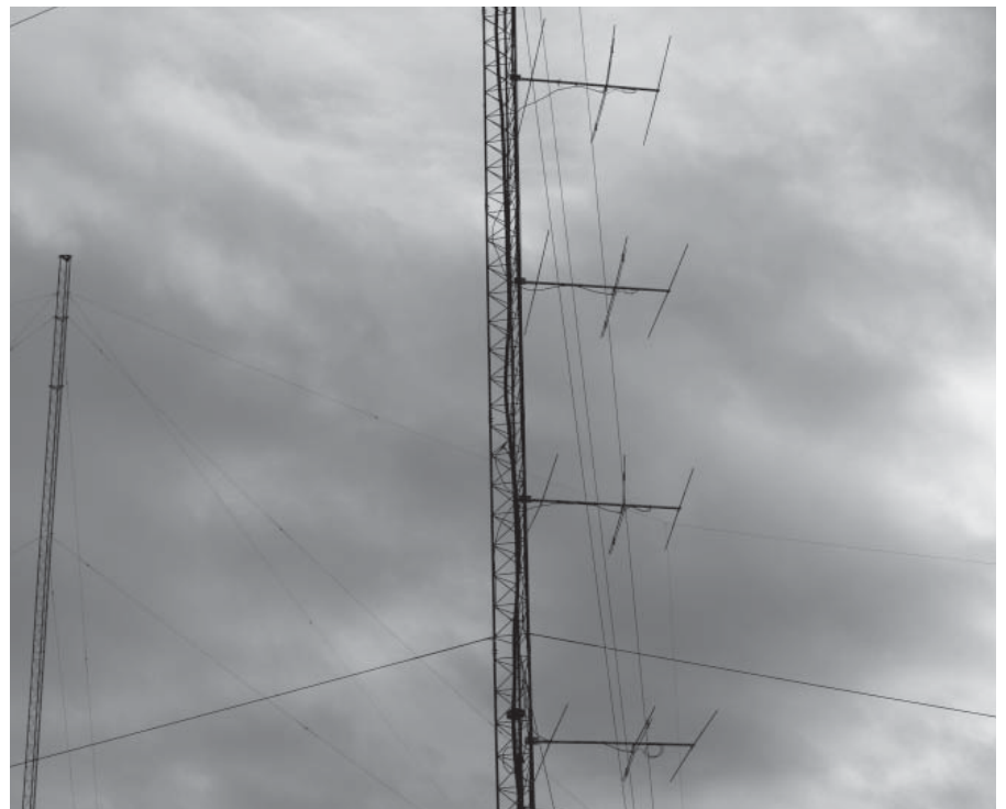
Figure 2 — A stack of four 3-element antennas for 50 MHz. These antennas have a 6-foot boom and are stacked approximately 10 feet apart. This array, with its small physical footprint, provides outstanding gain with an exceptionally low angle H-plane pattern and broad E-plane pattern.
