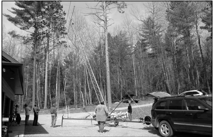
Fig 1—Correctly positioning the tower among the trees was a critical issue.
