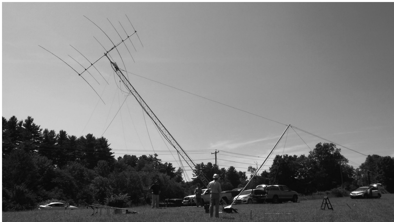
Figure 2 — An example of the falling derrick method being used to raise the tower and antenna [AE1P photo]
