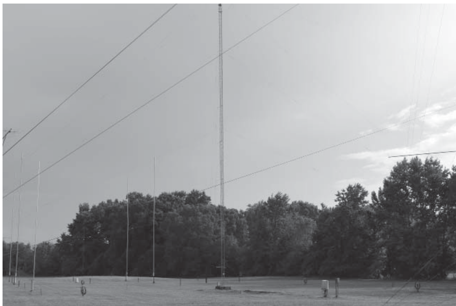
Figure 1 — The 160-meter driven element surrounded by the four parasitic elements.
