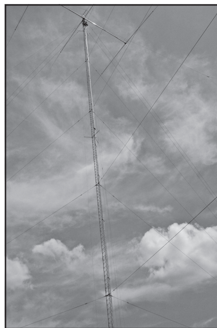
Figure 3—W5IZ's tower with the detuning skirt (you have to look closely to see the wires around the tower).
