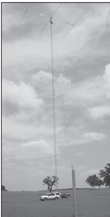
Figure 1—The 200 foot tower at W5IZ, with an 80-meter Yagi on top and a 4-Square system around it.
