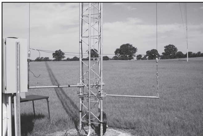
Figure 4—The insulated bottom of the skirt. Note the halo wires that tie the skirt wires together.
