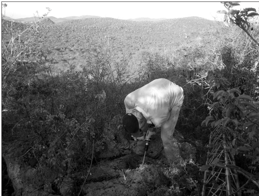
Some of the PJ2T challenges with antenna installation on a Caribbean Island: Goose Steingass, W8AV, drilling into solid rock.
