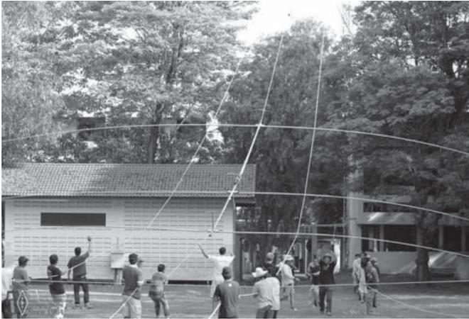
Figure 3 — In a big team effort, a homebrew 40-meter monoband Yagi is erected for HSØAC at AIT in June, 2014.
